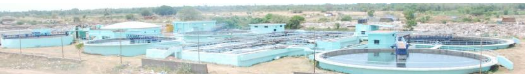
Birds-Eye view of the CMWSSB Kumbakonam Sewage Treatment Plant
